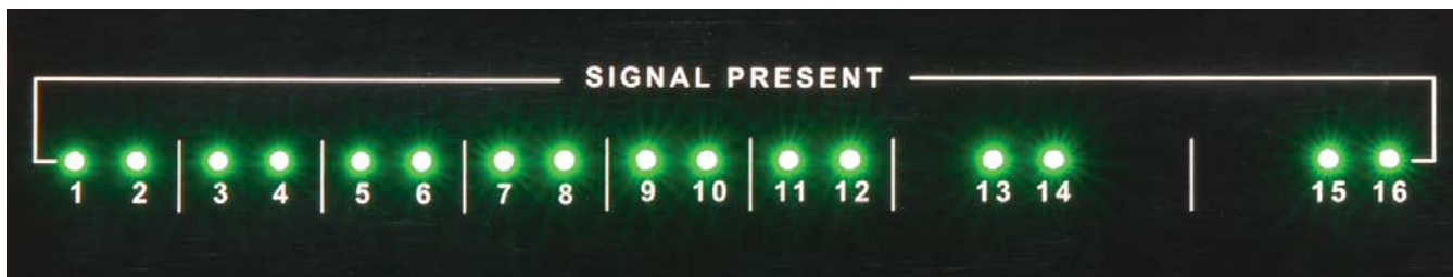
[SIGNAL PRESENT LEDS PICTURED ABOVE]
